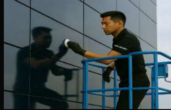
RENOVAR PANELES ACP
