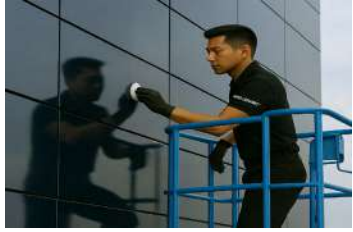
RENEW ACP PANELS
