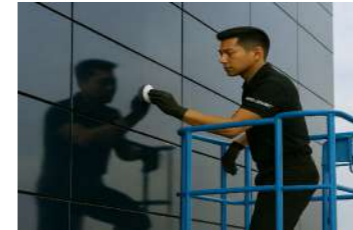
RENEW ACP PANELS
