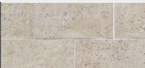
CRYSTALLISED LIME STONE
