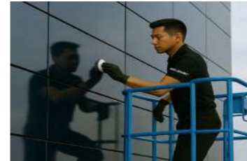
RENEW ACP PANELS
